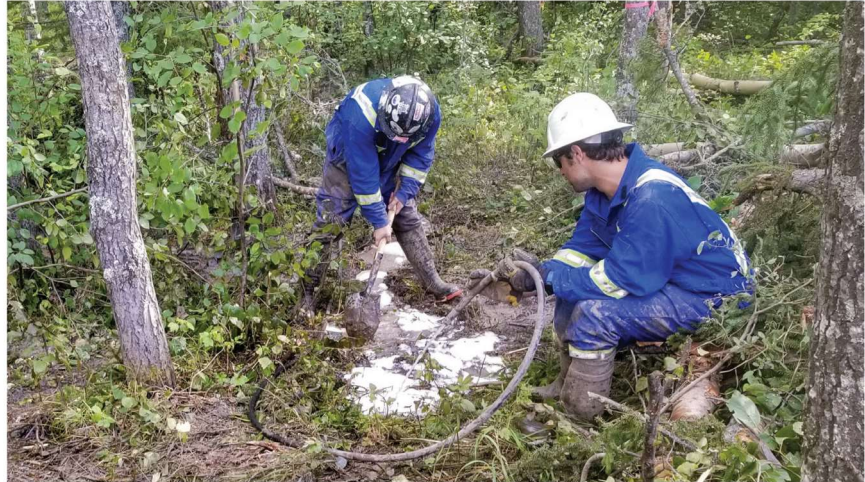
Cleanup crews flush forested impact site with Ivey-sol® surfactant.
