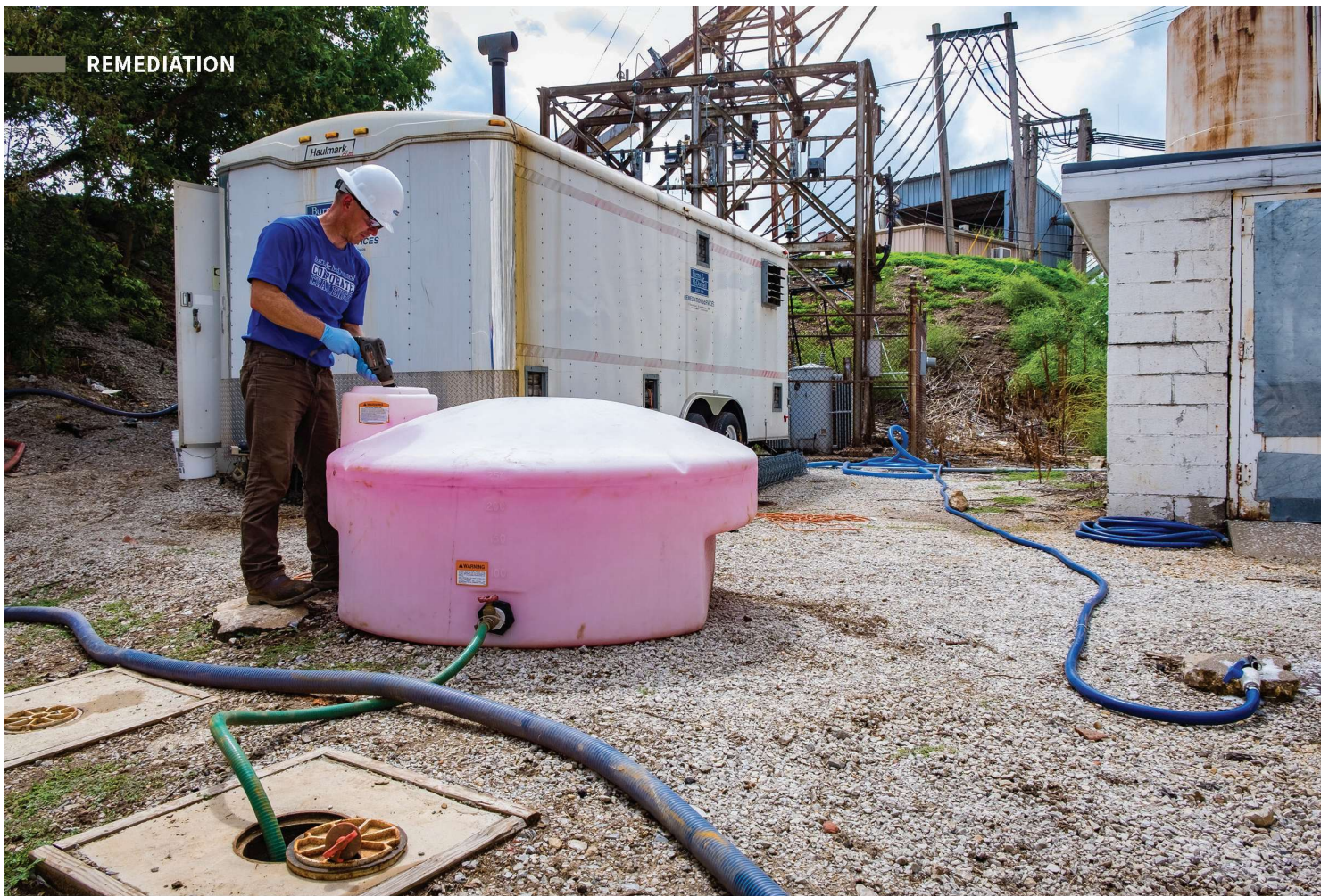
Ivey-sol 106 surfactant is mixed with water, with the addition of a conservative tracer for monitoring purposes, prior to injection.
